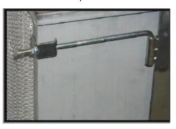
F. The preference is for filters to be loaded in the airstream and not slide out the side of the unit.
