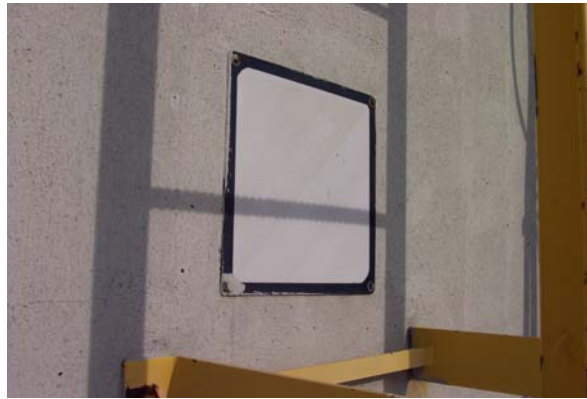
RF Sign Behind Ladder To Upper Roof
